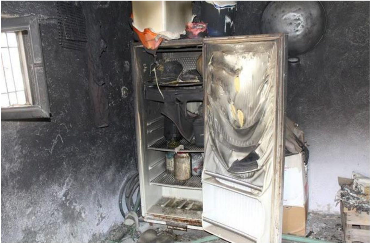
Photo: Kitchen of a house damaged during the curfew
