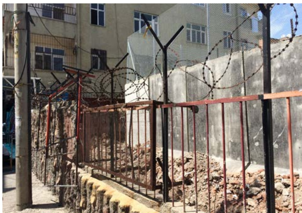
A health care facility in Diyarbakir's Bağlar neighborhood that was being turned into a police station, according to the Health Workers' Union (SES).
