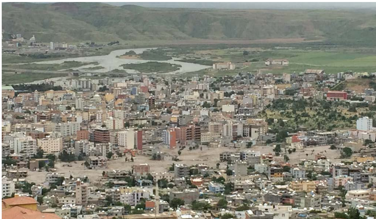
A view of Cizre showing the area where Turkish authorities razed buildings over a series of basements in which between 130 and 190 people were trapped for several weeks in the midst of heavy clashes and round-the-clock curfews. All of those trapped in the basements died.
