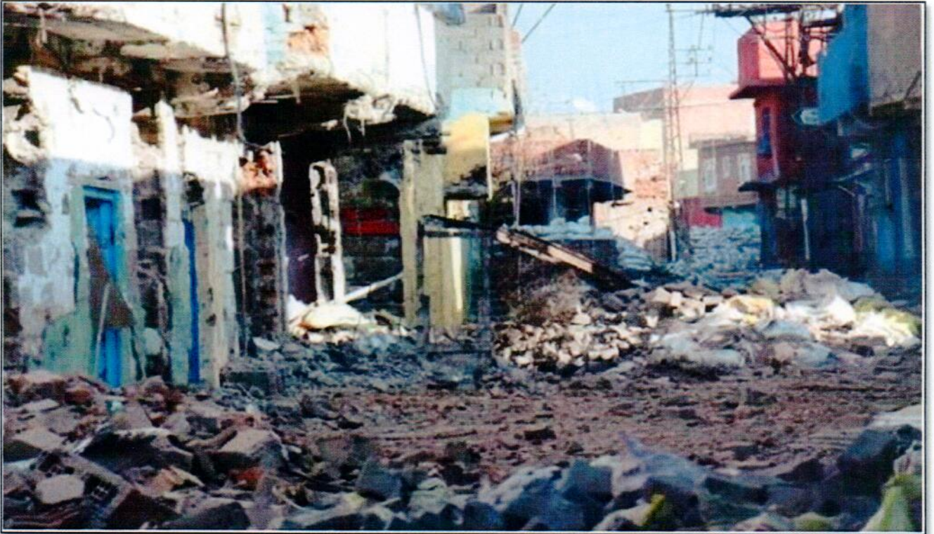
FOTO-6: HASIRLI MAHALLESİ- YIKIKKAYA SOKAK
